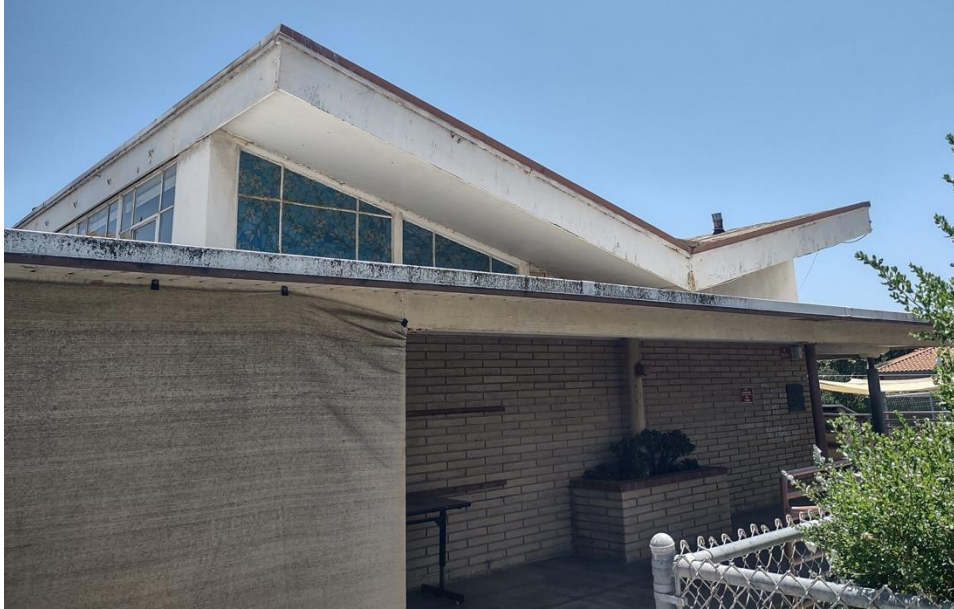
Photo 12 South Classroom Building, north elevation, view southeast; note steel frame, window wall, and CMU infill
