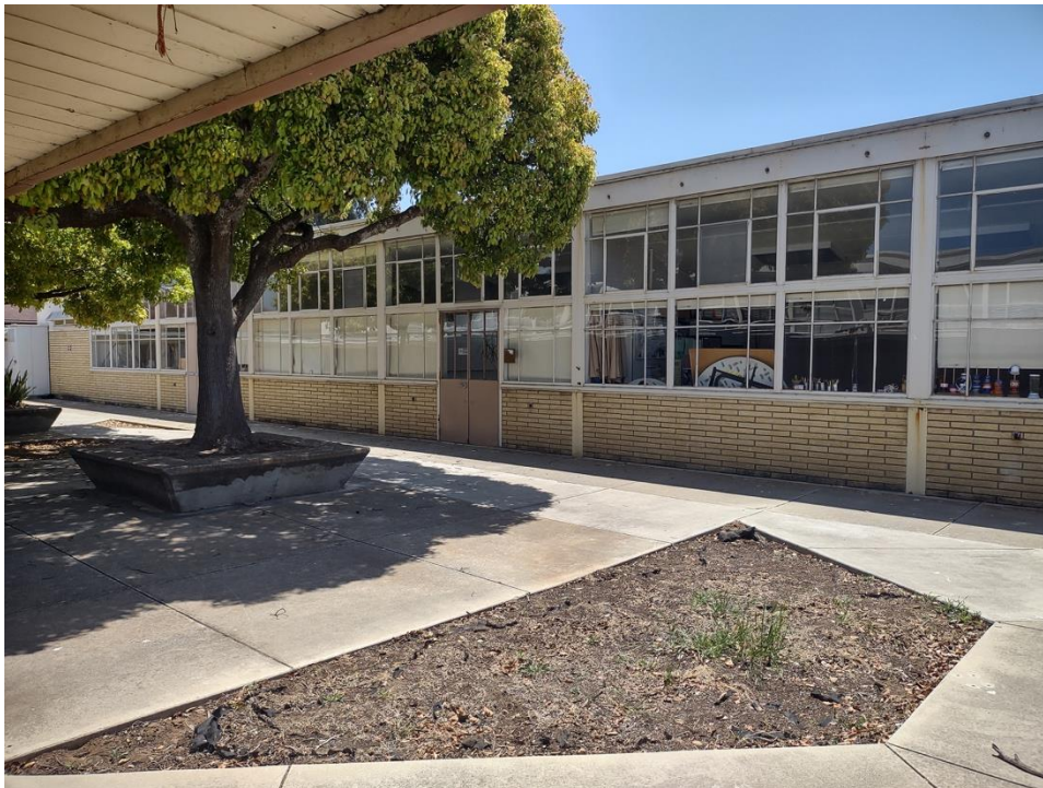
Photo 12 South Classroom Building, north elevation, view southeast; note steel frame, window wall, and CMU infill
