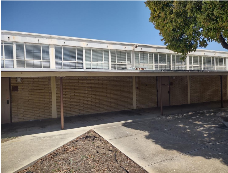
Photo 14 South Classroom Building, view showing V-shaped roof dip at interior, and exposed steel-frame and CMU wall
