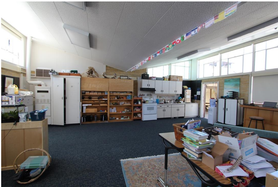
Photo 14 South Classroom Building, view showing V-shaped roof dip at interior, and exposed steel-frame and CMU wall
