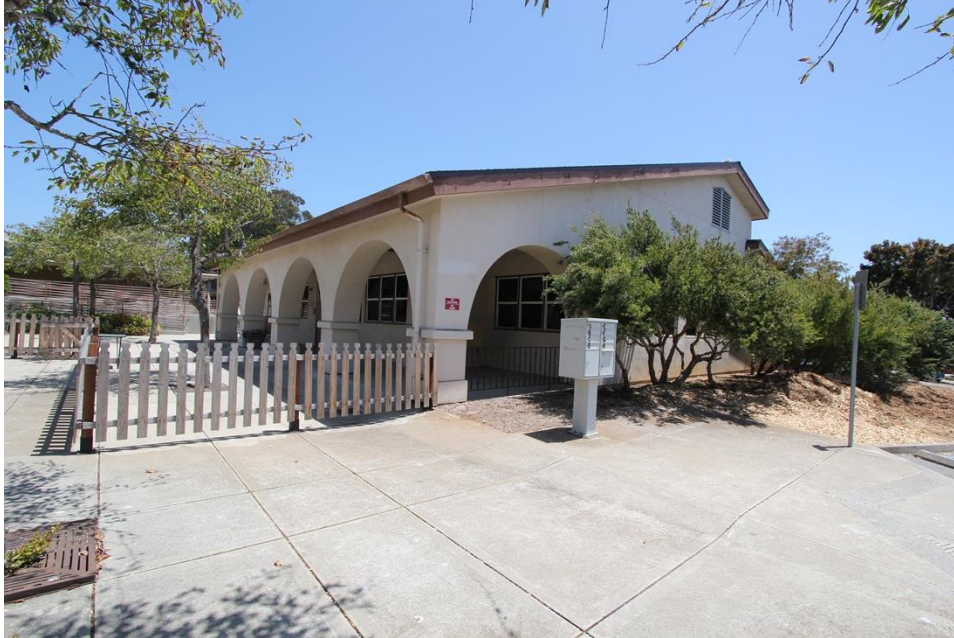
Photo 19 Charter School Building, west elevation (right) and north elevation (left), view southeast
